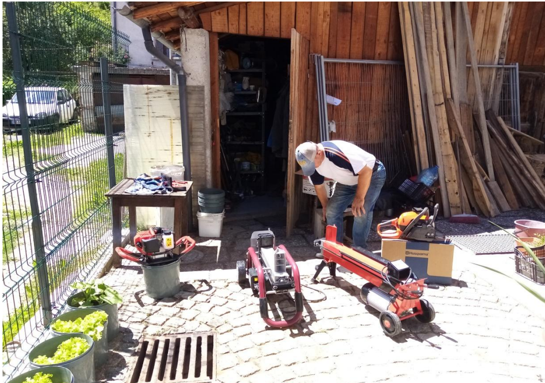
Inspection and preparation of delivery machines before forthcoming work
